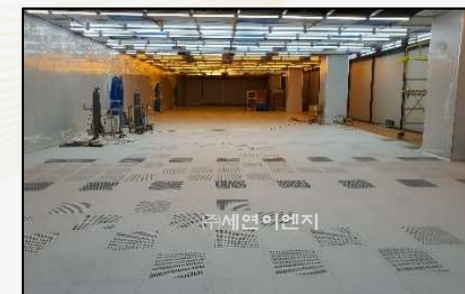
ACCESS FLOOR PANEL 설치
